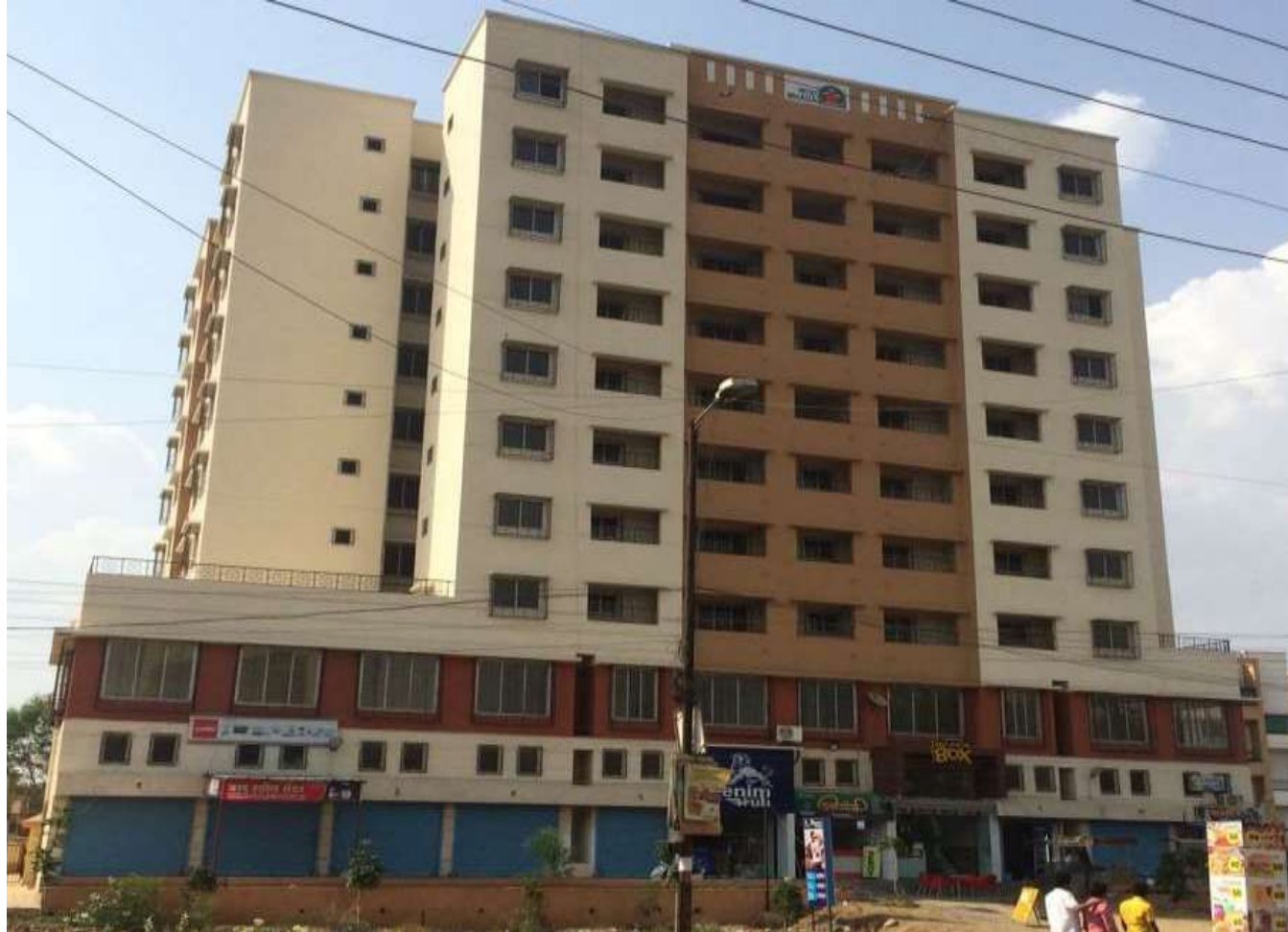
SPA-I Solapur (Near D Mart)
